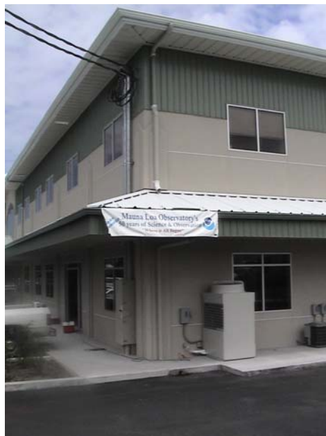
Banner in front of the building.
